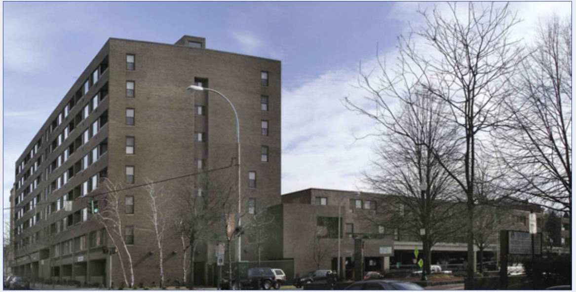
Peekskill Plaza has seen major improvements inside and out, including new appliances in its rooms, repair of leaks and brickwork, and improvement of its retail spaces.
