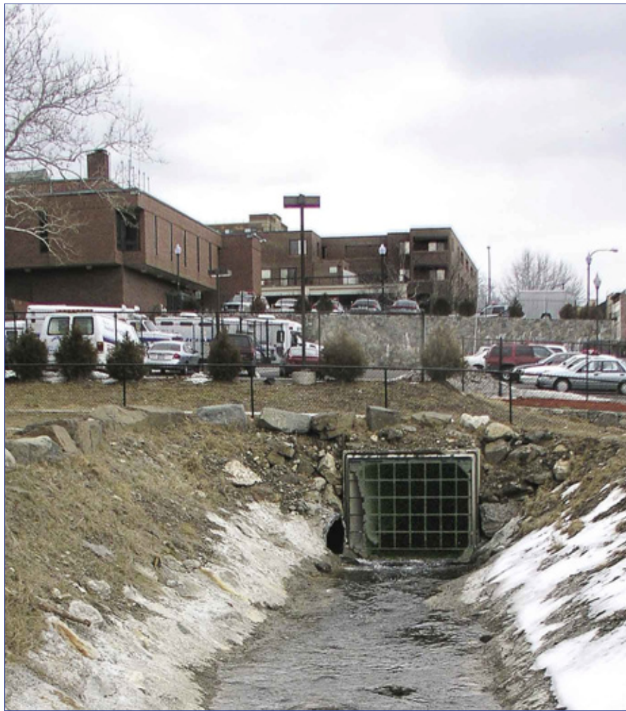
Five achievements are embodied in this image. A new park with brook is created, a new police parking lot is built and another expanded, flood control is increased significantly, and FEMA pays for most of the work.
